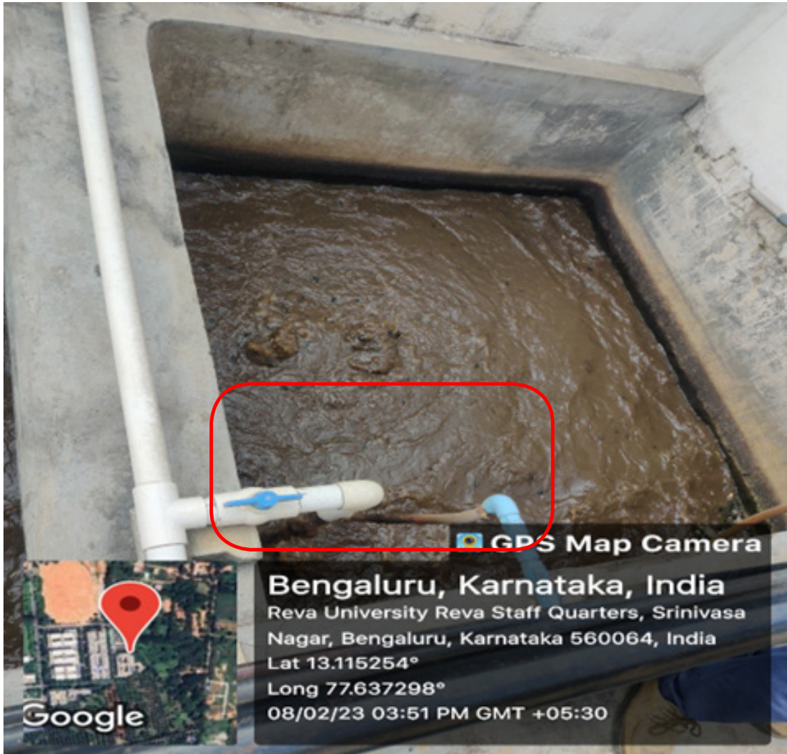
Wastewater treatment unit after pumping Block: Sewage Treatment Plant, REVA University
