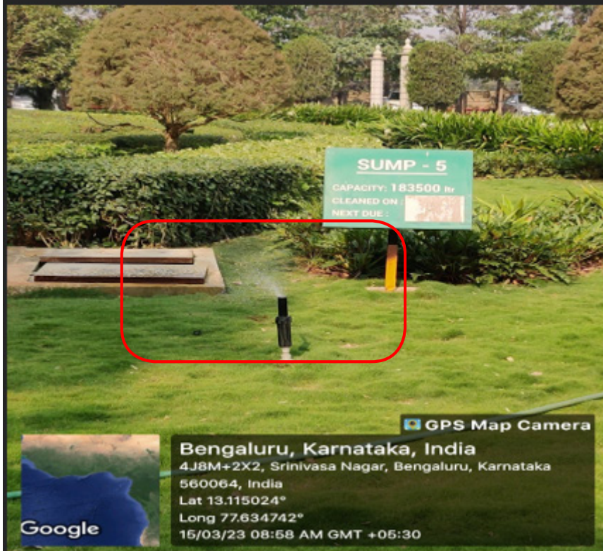
Water distribution through sprinkler Block- REVA Admin Block
