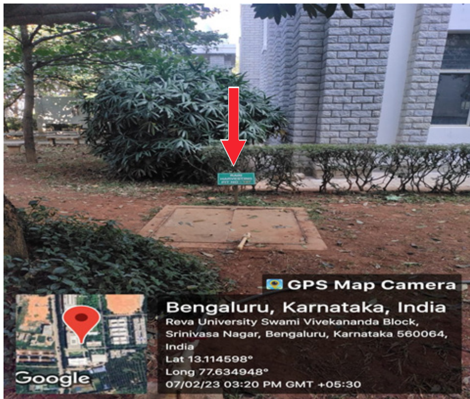
Rainwater reservation pits and labels Location: Throughout the REVA University Campus
