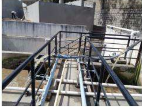
← Sewage Treatment Plant
