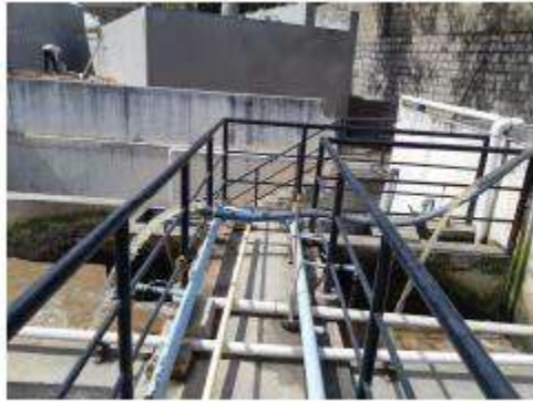
← Sewage Treatment Plant
